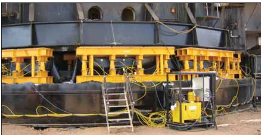
◀ Shown: Dragline joint separation using Enerpac Synchronous Lifting System.
